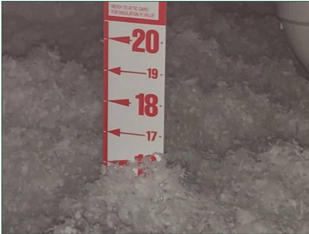
Figure 10. Measuring Stick Aiding in Observation of Blown in Insulation
