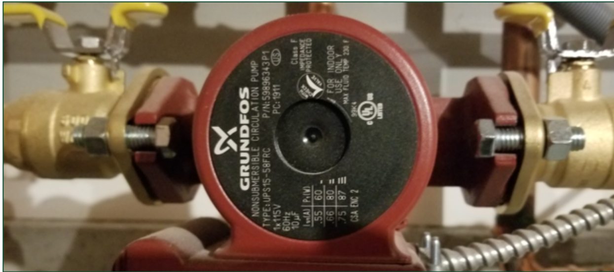
Figure 72. 3-Speed Hydronic Circulation Pump
