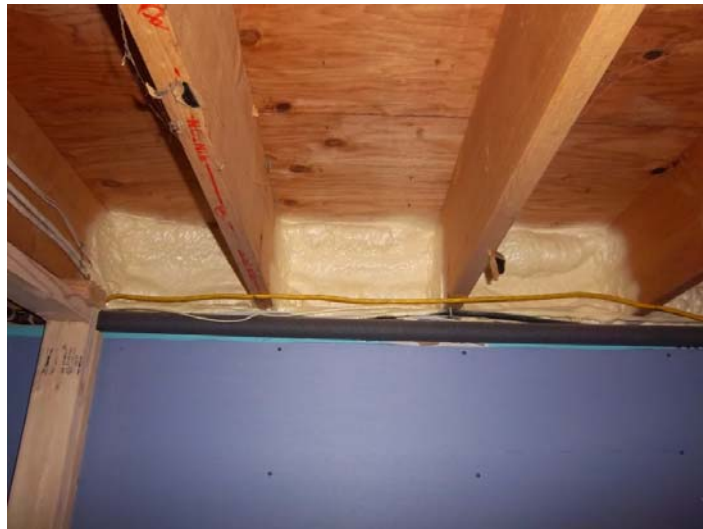
Figure 17. Rim and Band Joist Insulation
