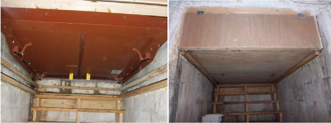
Figure 15. Basement Bulkhead Doors
