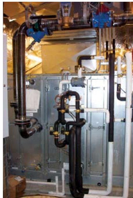
High-efficiency air handling unit at the Lincolnville Central School.
