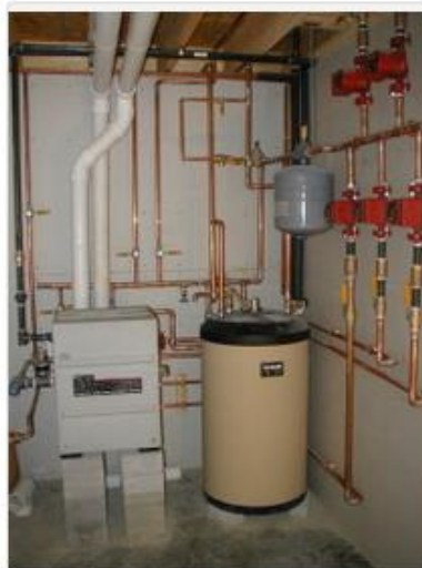
High-efficiency boiler with domestic hot water tank.
