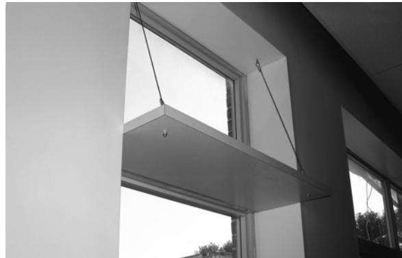
This panel reflects daylight onto the ceiling reducing the amount of artificial lighting needed
