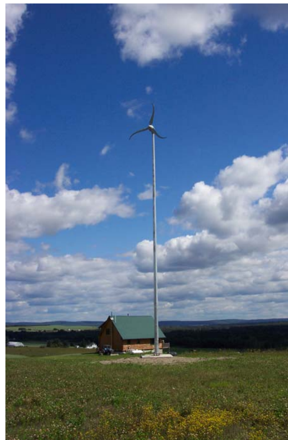
Installed by Green Earth Energy, Fort Kent
