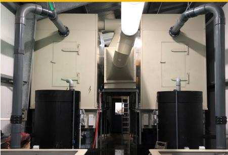
Using **\$130,000 in incentives** from Efficiency Maine, American Unagi installed two value-added equipment options that have reduced facility energy costs and lowered the farm's carbon footprint: **High-efficiency oxygenation equipment** delivering oxygen during water pumping and **specialized energy recovery ventilators** which are designed to operate in the high humidity conditions of indoor aquaculture.
