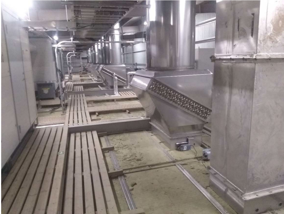
Attic Kiln with Heat Recovery Coils (Lumber processing facility)
