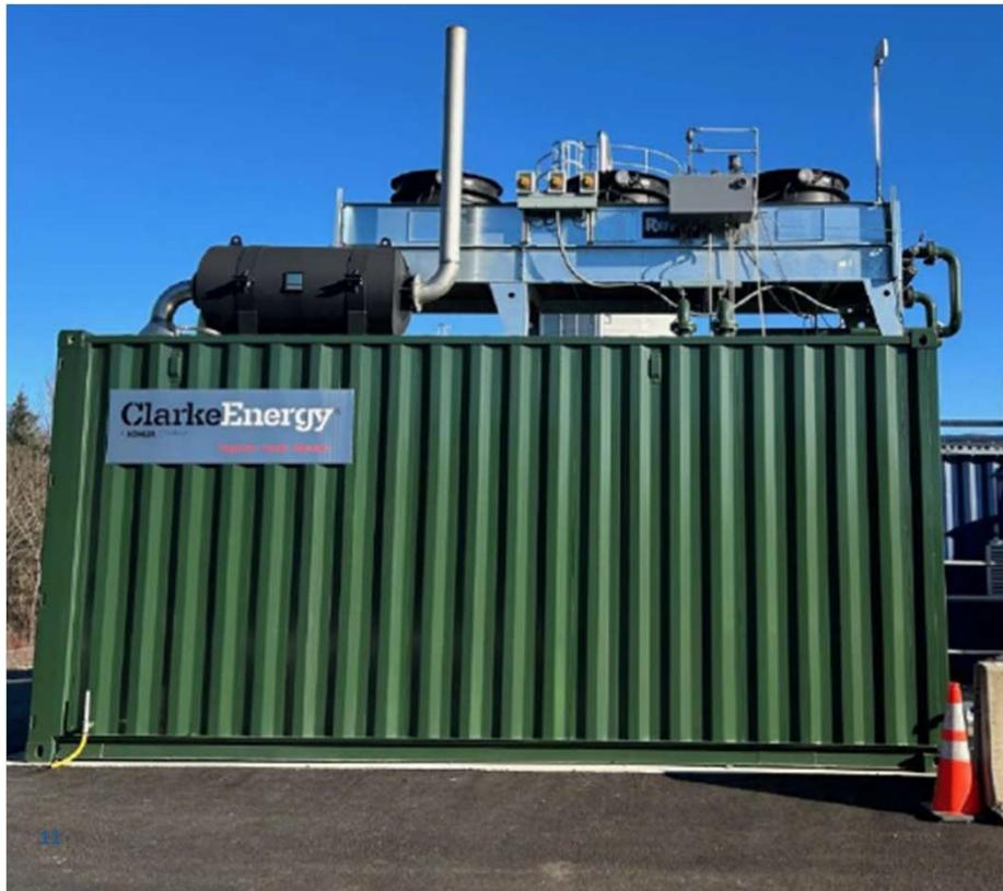
Peaks Renewables is a renewable energy development company that recently completed an anaerobic digester facility producing pipeline quality natural gas from cow manure on the Flood Brother's farm in Clinton. Custom supported a 280-kW combined heat and power unit onsite that serves digester thermal and electric loads.
