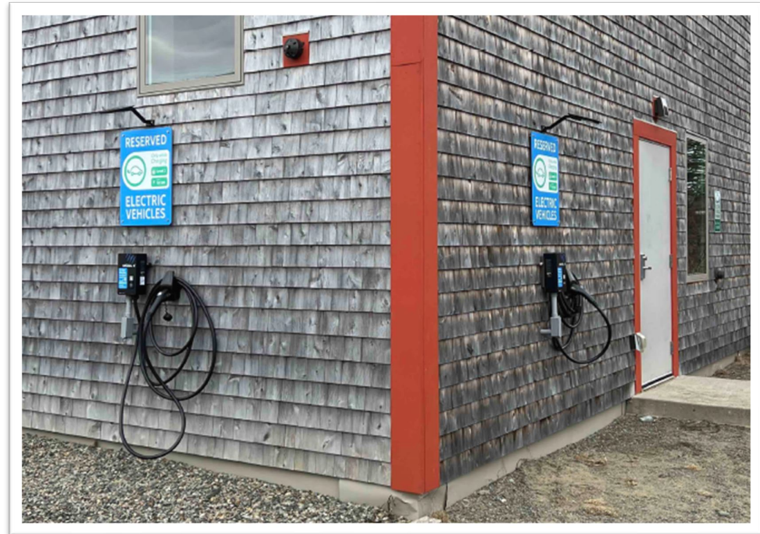
Cobscook Institute level 2 chargers in Lubec
