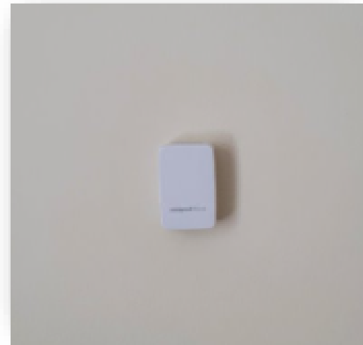
A mid-wall thermostat for a transfer fan.
