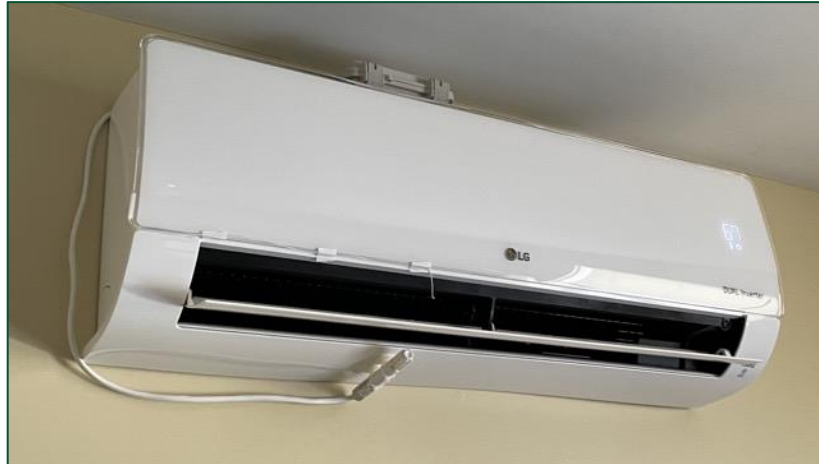
Figure 16. LORA Node Humidity Sensor and Thermistor on an Indoor Unit
