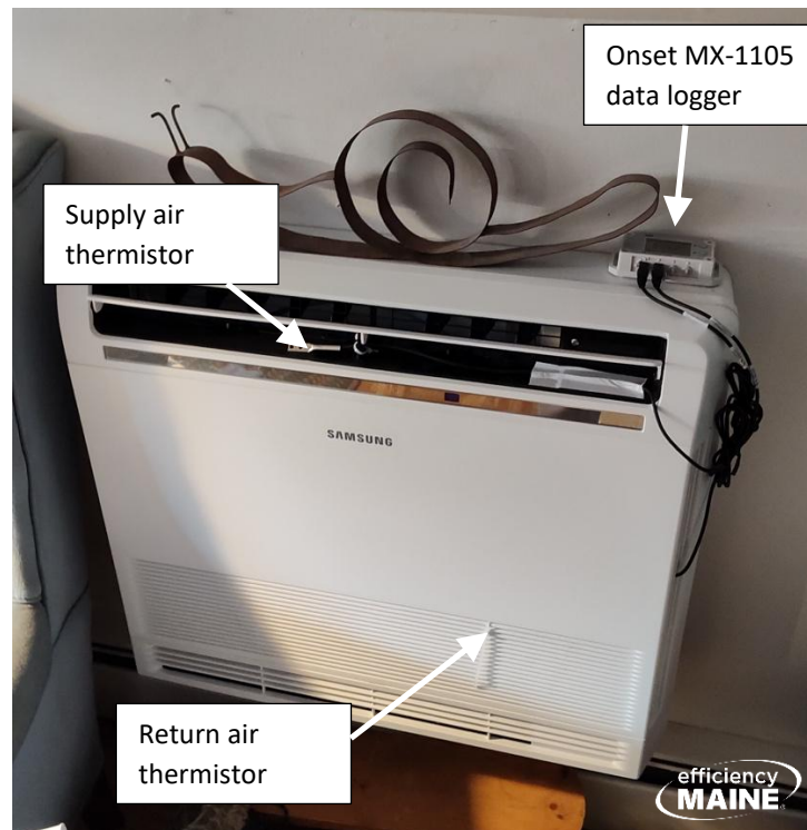
Figure 96. Thermistor and Logger on an Indoor Unit to Meter Supply and Return Temperatures
