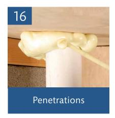
There can be gaps where any plumbing or electrical work runs through exterior walls and between floors. These gaps could allow air to flow between unheated and heated spaces. Consider sealing all holes with spray foam sealant or caulking to stop air movement.
