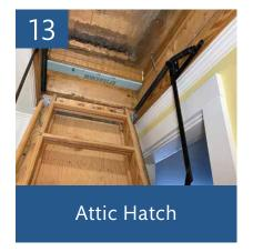
If you have pull-down attic stairs or an attic door, consider sealing it: weather strip the edges and put a piece of rigid foam board insulation on the back of the door. Treat the attic door like a door to the outside. Pre-made insulated attic stair covers are also available from local home-improvement centers or online.
