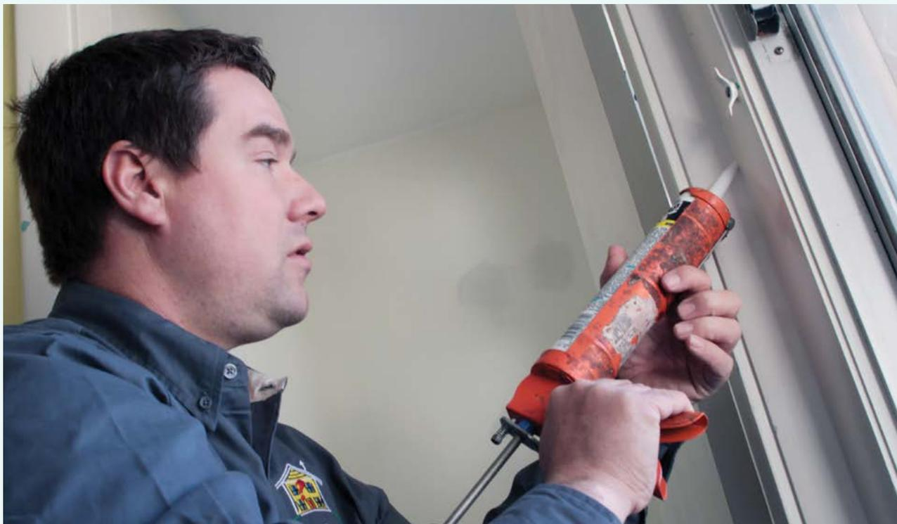
Does your home suffer from ice dams, frozen pipes, or cold spots? Are you tired of wasting money to heat a leaky home? Weatherization may address these problems and deliver increased year-round comfort. Weatherization involves air sealing and increasing the insulation in your attic, basement, and walls.
