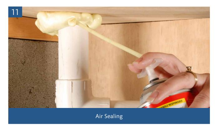
Air sealing reduces drafts and heat loss by eliminating air leaks in your home. Professional air sealers use a variety of materials, including caulk, spray foam, metal flashing, weather stripping, and rigid foam. Some materials are more suitable than others for specific locations or trouble spots. For example, fire-rated caulk and metal flashing are used around the chimney and in other high-temperature air-sealing situations.
