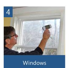
Insulating windows around their edges makes your home more energy efficient. To reduce heat loss in winter, install storm windows, transparent plastic window film, or indoor window inserts. When purchasing windows, look for ENERGY STAR-certified models designed for Maine's climate.
