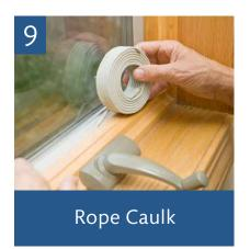
Consider installing a temporary seal around windows and doors that won't be used for long periods of time, such as a basement door that is unused in the winter. Many types of rope caulk can be easily removed in the spring and stored in a plastic bag for reuse the following season. To fill larger gaps, use several strands twisted together.
