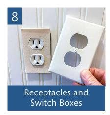
Seal outlets and switch boxes with foam gaskets. Installing foam gaskets can reduce drafts and create an extra barrier between warmer and cooler air.
