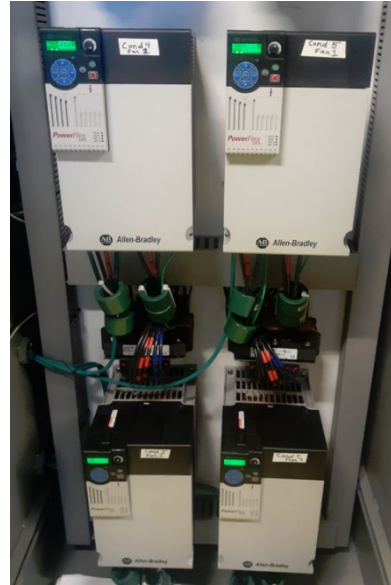
Photo 2 – VFD Controllers
