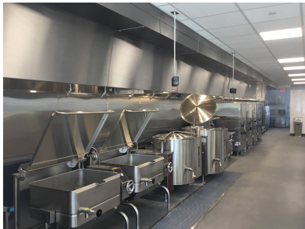
Kitchen Exhaust Hoods with EcoAzure Demand Controls
