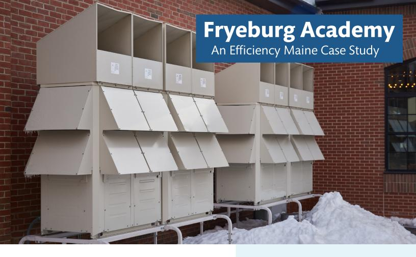
Efficiency Maine worked with Fryeburg Academy to install two VRF systems with heat recovery in their campus student union building. VRF systems are a highly efficient heating and cooling technology for larger buildings, and have the ability to simultaneously heat one space while cooling another.
