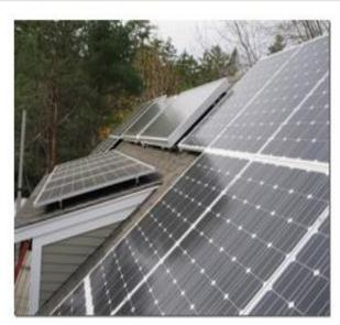
A typical solar electric system is an array of solar modules or panels, mounted on racks and connected to the utility grid or to batteries through a power inverter. The performance of photovoltaic or solar electric systems is measured in terms of their efficiency at converting sunlight into electricity. There are a variety of solar electric systems and materials available, which vary in conversion efficiency.
